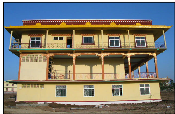
New Gompa in final phase of construction.
