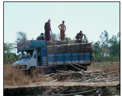
Monks unloading trucks with materials for building the Gompa.
